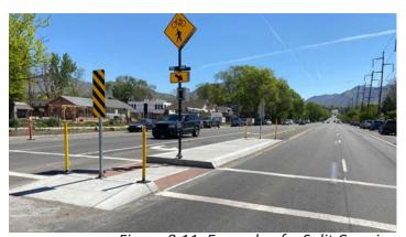
Figure 8.11. Example of a Split Crossing Source: Salt Lake City Transportation
