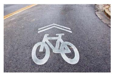
Figure 8.22. Shared Roadway Marking or "Sharrow" Source: BikeTexas
